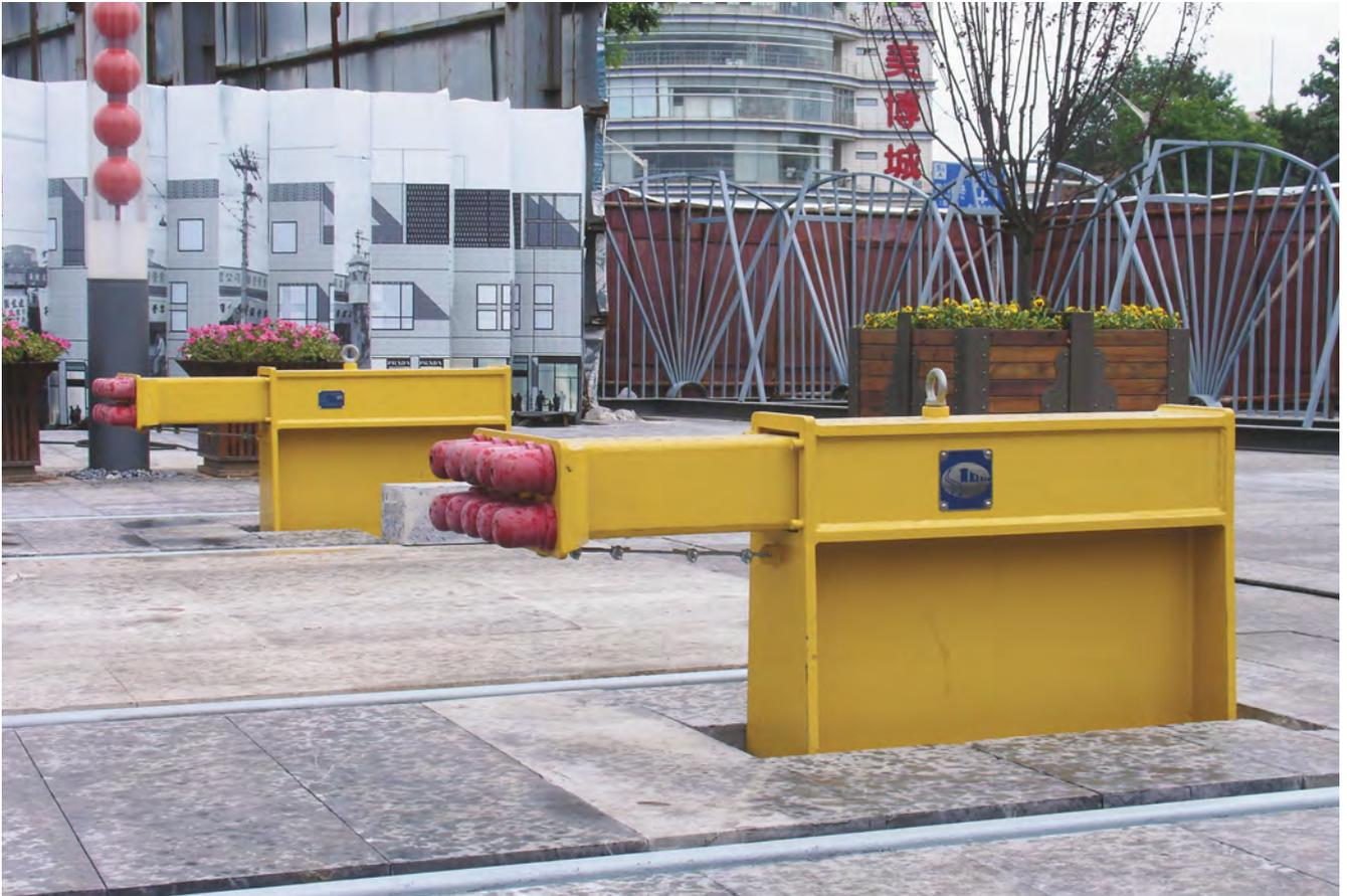
This end stop was designed to support a specific rebuilding project to create an old style tram in Beijing – designed for centre impact with rubber softener. Fixed end stop incorporating Oleo hydraulic unit (one Type 54 – Recoverable stroke 400mm). Impact capacity: 160kJ.
